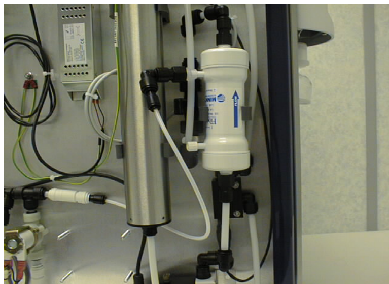
Fig-18 Location of Internal (0.2/0.05um) Filter
